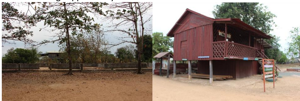
Figure 1: (a) An old school building destroyed by the storm; and (b) The new school building supported by United World Schools
